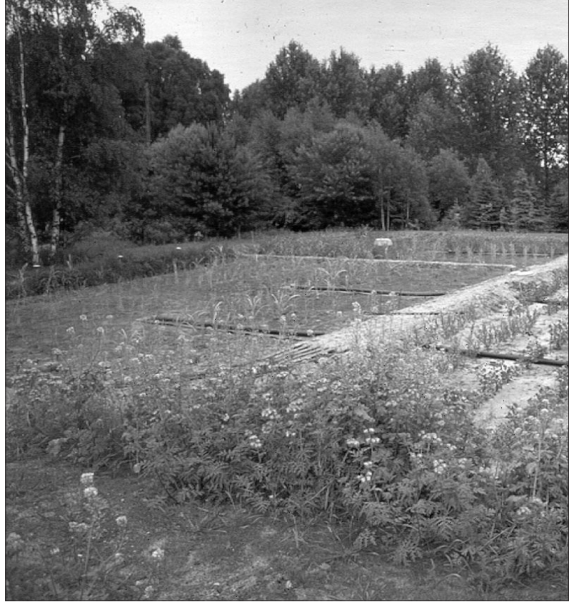
Water purification plant at the time of construction 1992.
